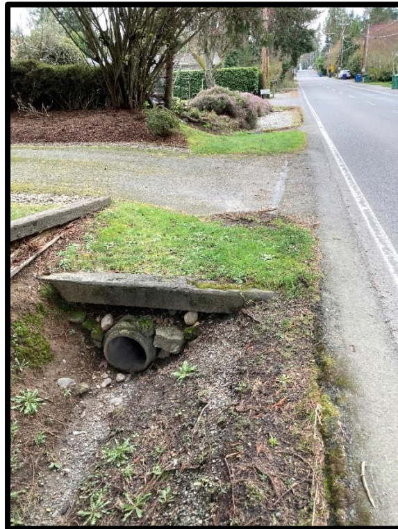
Element D: 8" concrete culvert along eastern side of 72 nd Avenue SE
